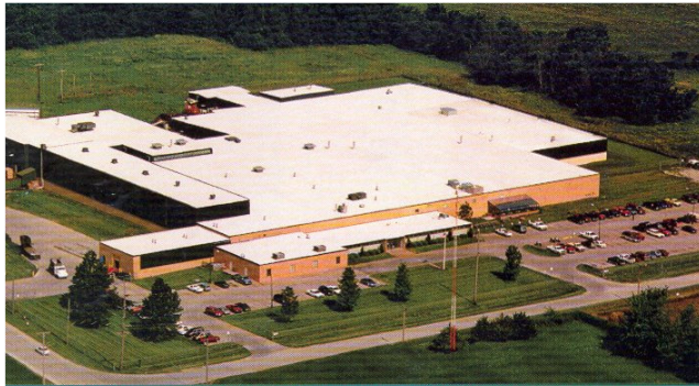
237,000 sf industrial facility available in Fairfield, Iowa
